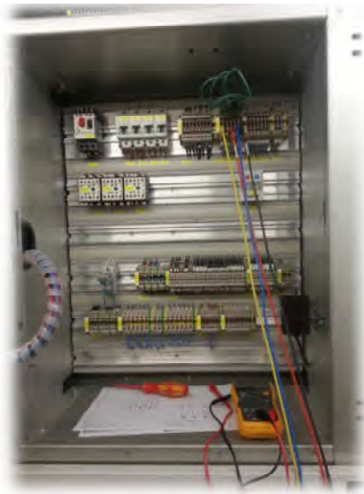
Commissioning of MM200 motor protection relays in Los Guinchos Power Plant (La Palma – Canary Islands) Spain
